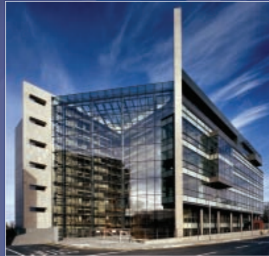
Central Park, Leopardstown, Dublin. Tegral Composite Floor Decking
