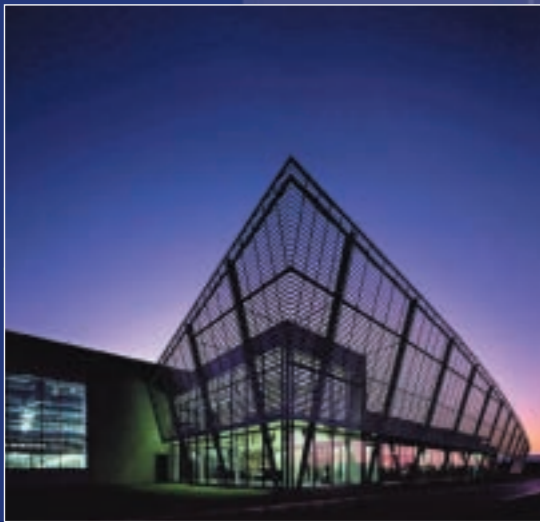
Bailey's Production Facility, Mallusk. Tegral Twin-Skin Roofing and Cladding
